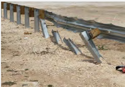
Guardrail damage resulting from MASH Test 3-10 in Test No. 420020-5.
